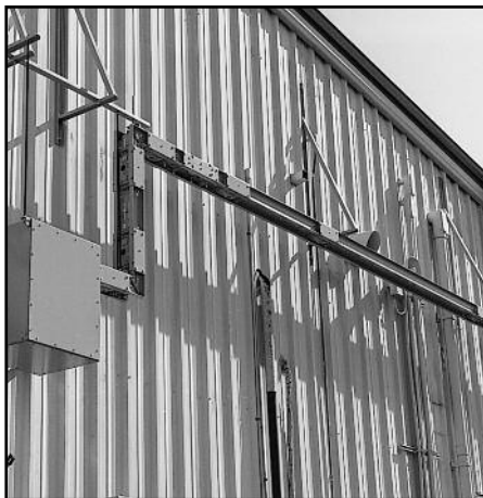
Complete outdoor run of Spectra Series busway.
